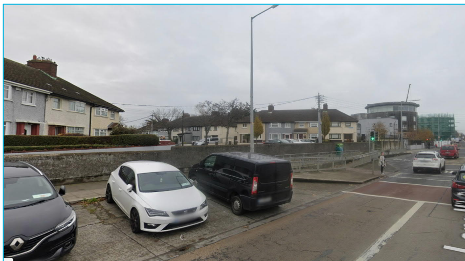
Figure 8-3 RW03 Long Mile Road Retaining Wall
