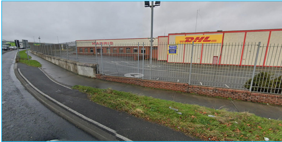
Figure 8-4 RW04 Naas Road Retaining Wall No.1
