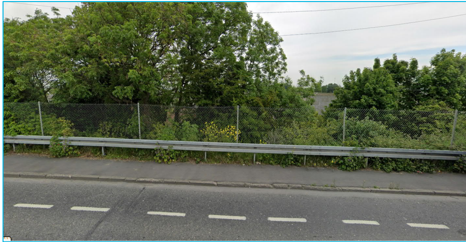
Figure 8-1 RW01 Calmount Road Retaining Wall No.1
