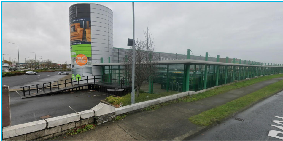
Figure 8-5 RW05 Naas Road Retaining Wall No.2
