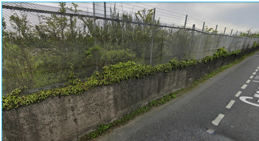
Figure 8-2 RW02 Calmount Road Retaining Wall No.2
