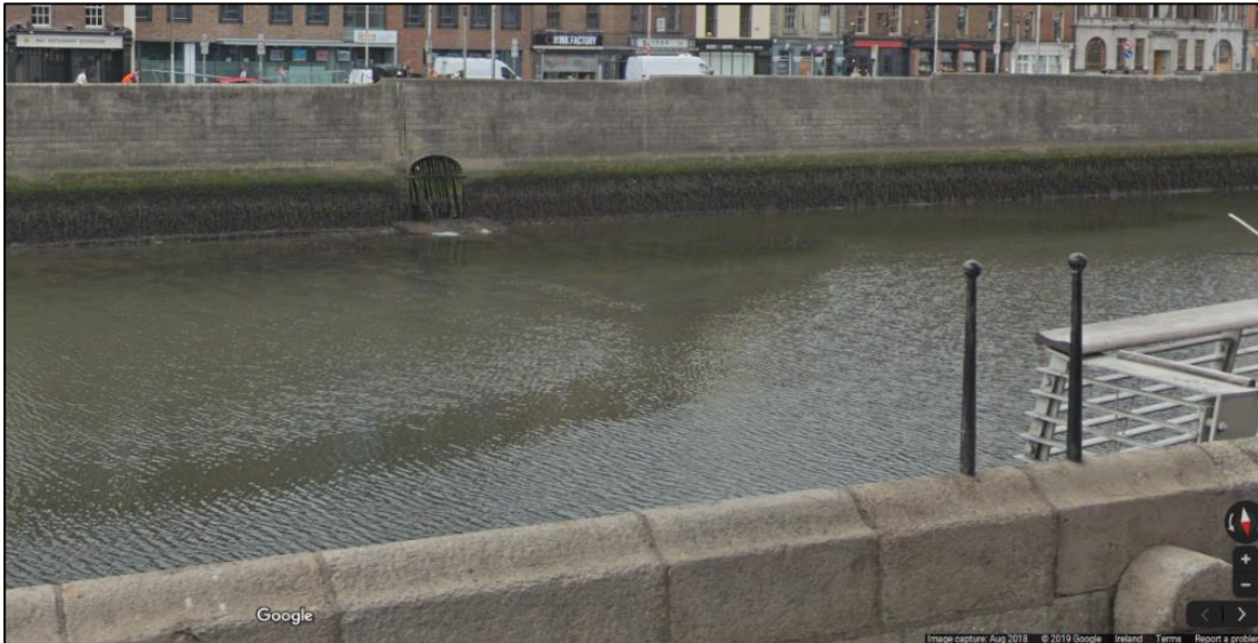
Figure 16: River Poddle Outfall to the River Liffey
