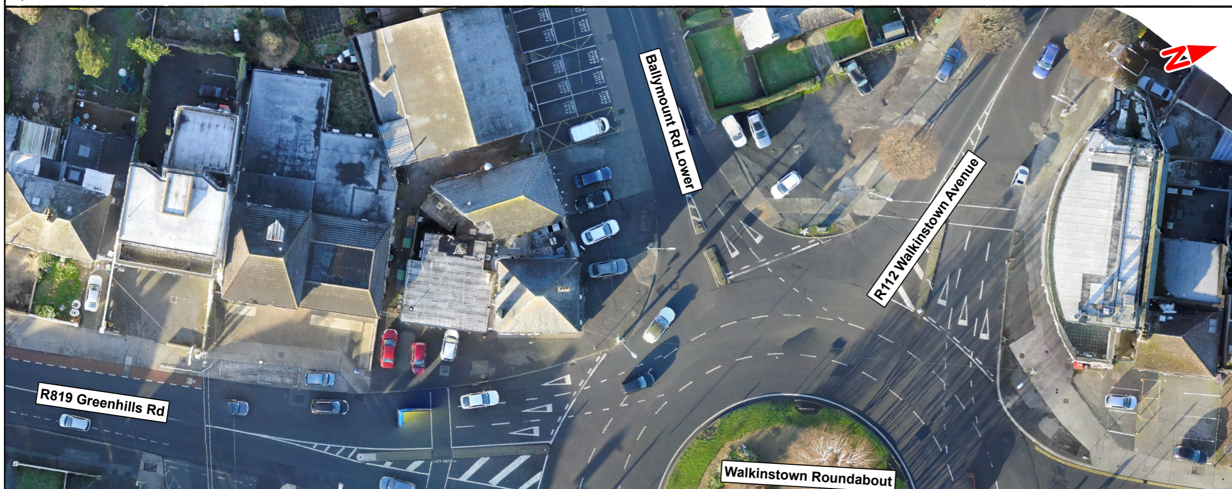
B) WALKINSTOWN ROUNDABOUT NORTHERN SECTION
